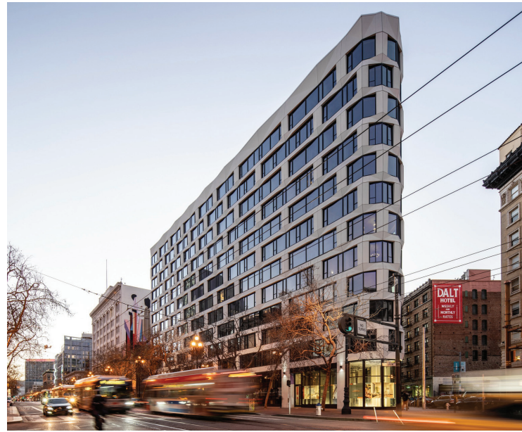
Serif Residences and the Line Hotel in downtown San Francisco used 671 precast concrete panels made of 79,000 ft 2 (7300 m 2 ) of glass-fiber-reinforced concrete. Courtesy of Jason O'Rear Photography.
