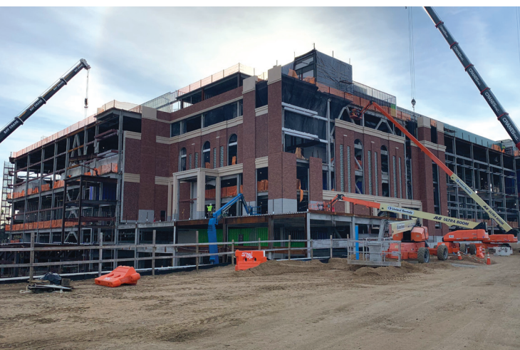
The new UBS Arena in Nassau County, N.Y., home of the New York Islanders professional hockey team, was designed with thermal performance and reduced energy use in mind. Precast concrete helped meet these requirements through the use of continuous, edge-to-edge insulation. Courtesy of Elizabeth Strohl.
